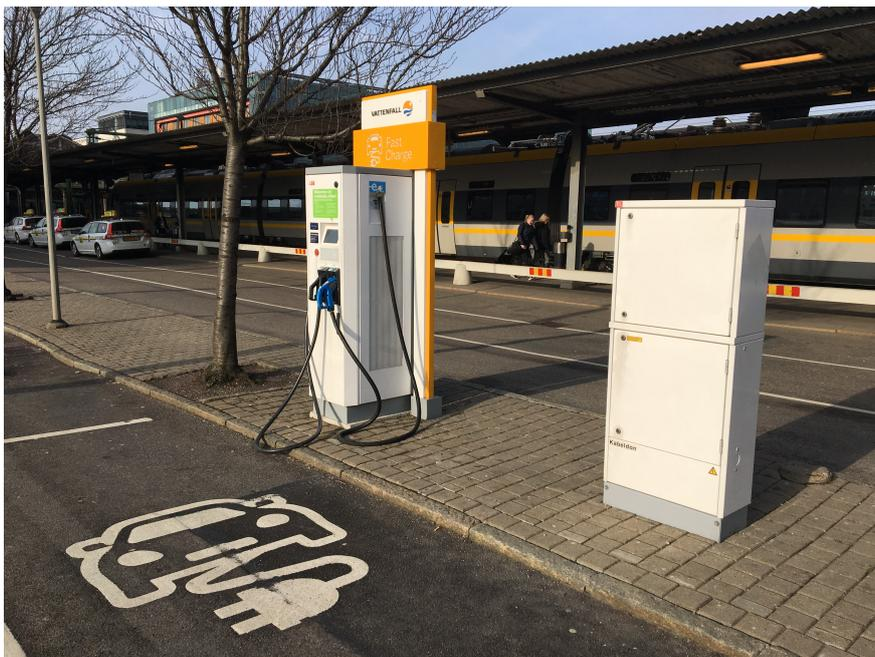
Figure A.2: CDC feeding an EV charger (ABB, 2019b)
