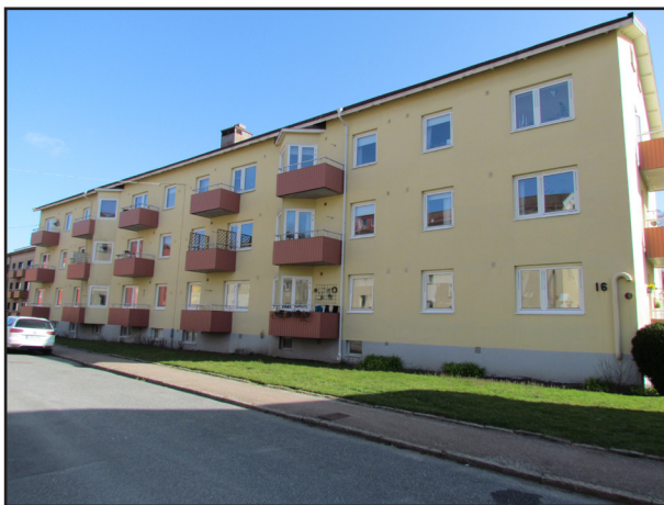
Figur 6: Fastighet i Torp
