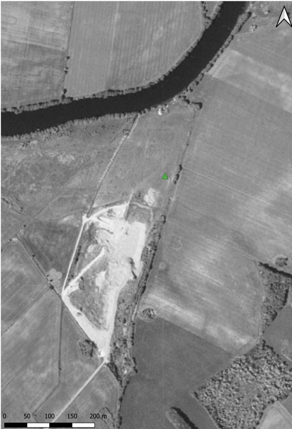
Figure 26. Orthophoto over the area H19031, marked with a green triangle) from the year 1975 before the restoration.
