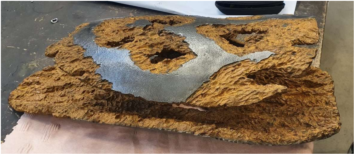
Figure 29. Before surface treatment, Halkosaari, 2020
