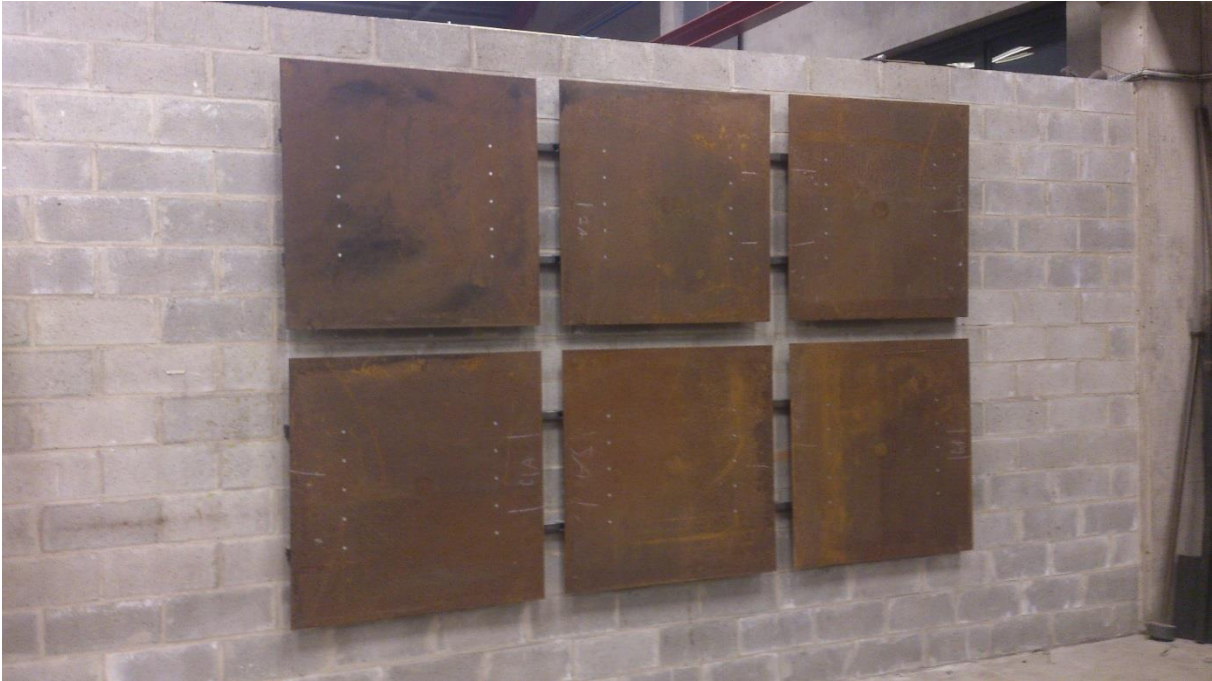
The panels mounted on the wall, total dimension 3.20 x 2.10 m.
