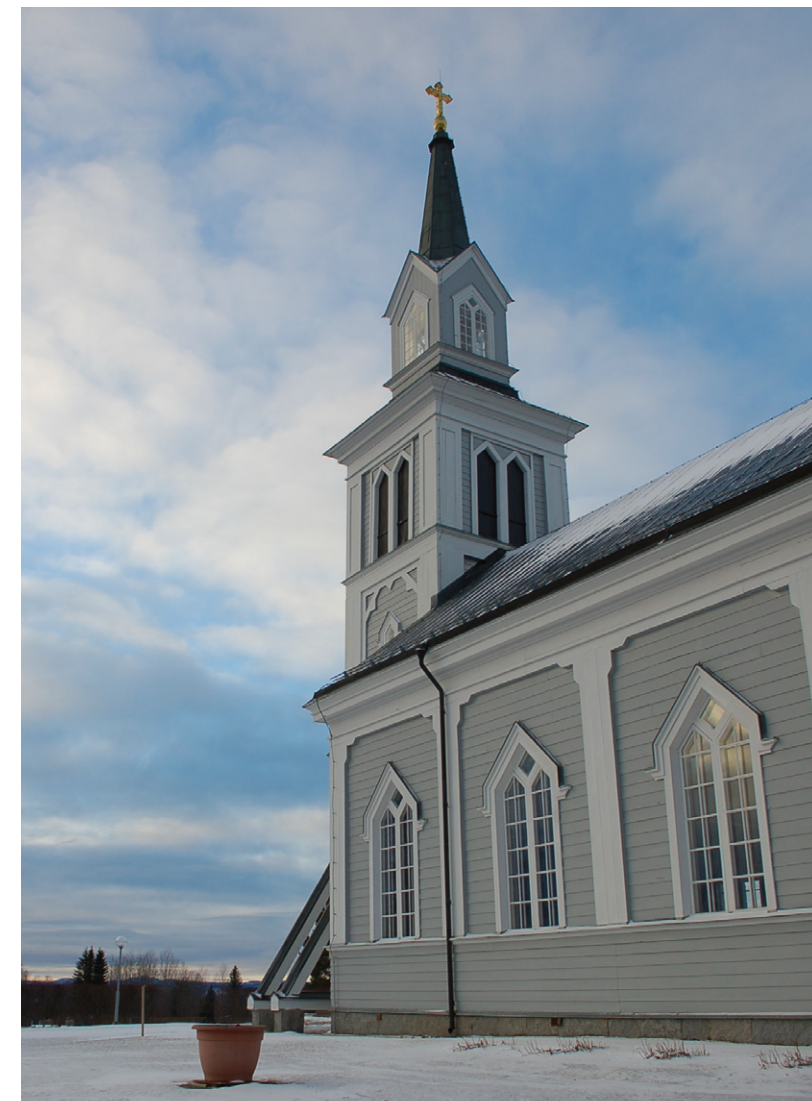
Figure 5. Hamra Church seen from the south in November 2017. Photo by author.
