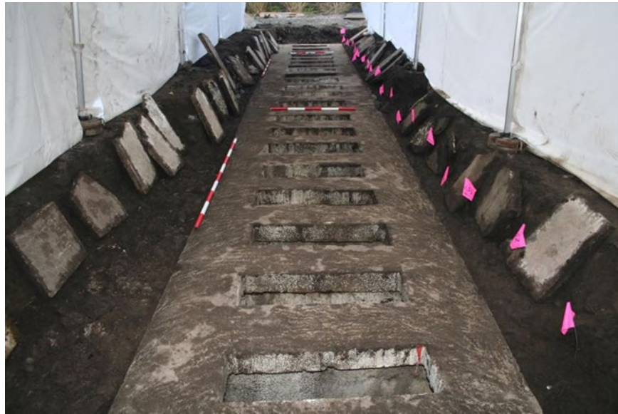
Figure 11 Picture taken from phase IIA of the tanks with the concrete lids removed (MBHCOI 2019b Appendix C 2017)
