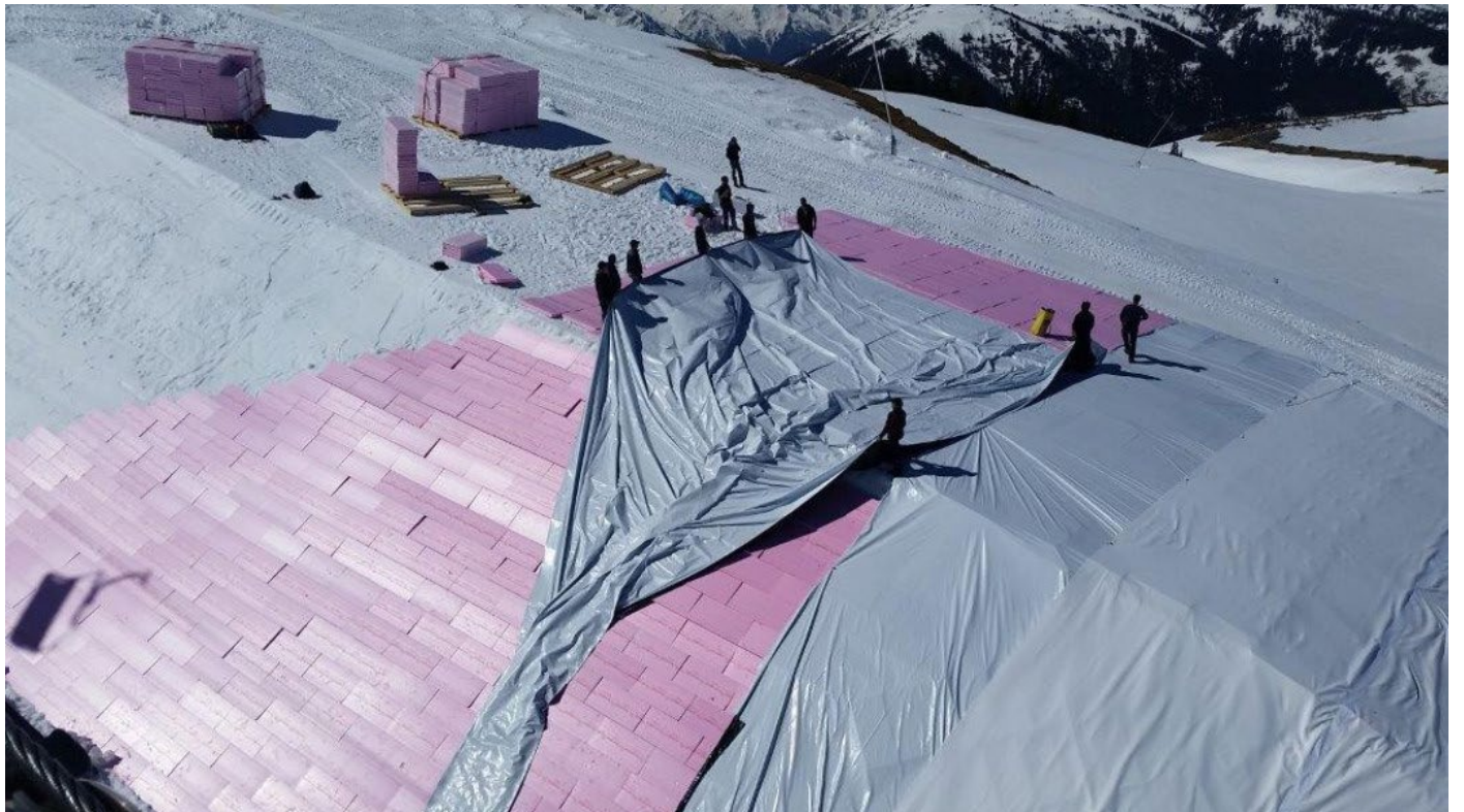
Kitzbühel, snow depot covered in foamboards and foils, ©Bergbahn AG, Kitzbühel
