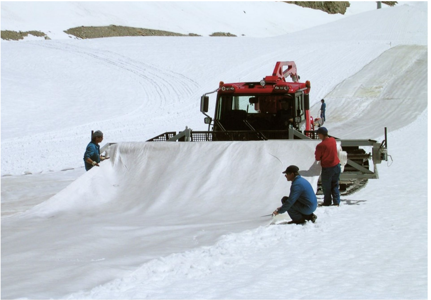
— Workers cover the ski slopes on the Pitztal Glacier in Austria with an innovative white fleece in an effort to protect the mountain from glacier
